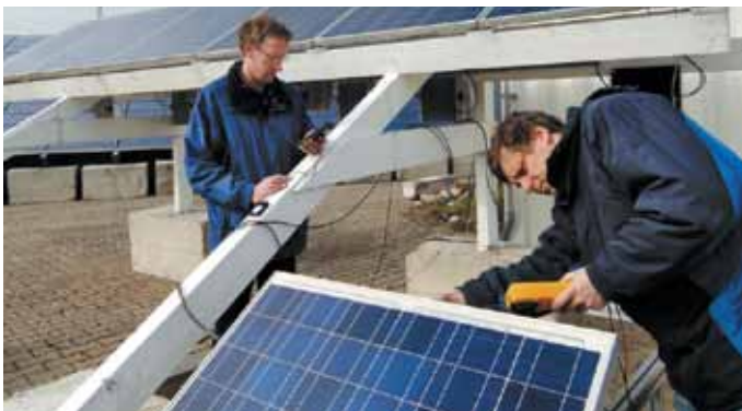
Installation of Photon Lab's outdoor module test. Photo: photon-pictures.com
